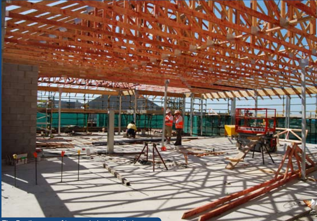
The Boathouse roof trusses being installed
