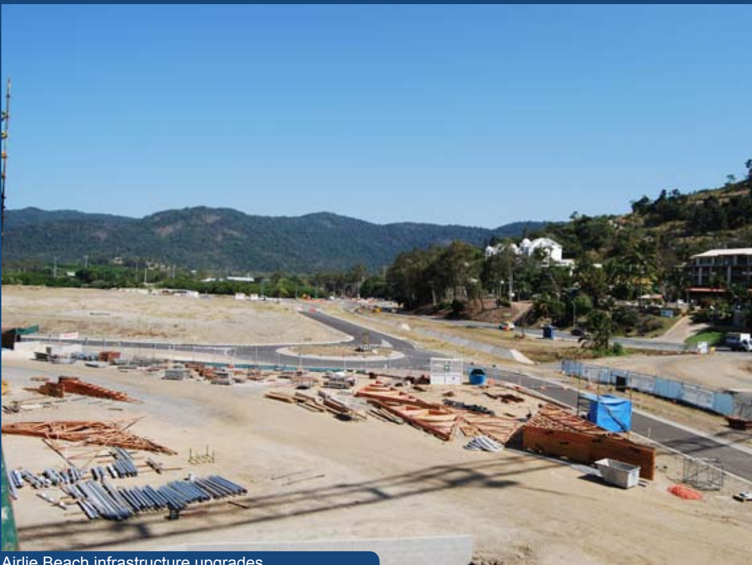
Airlie Beach infrastructure upgrades
