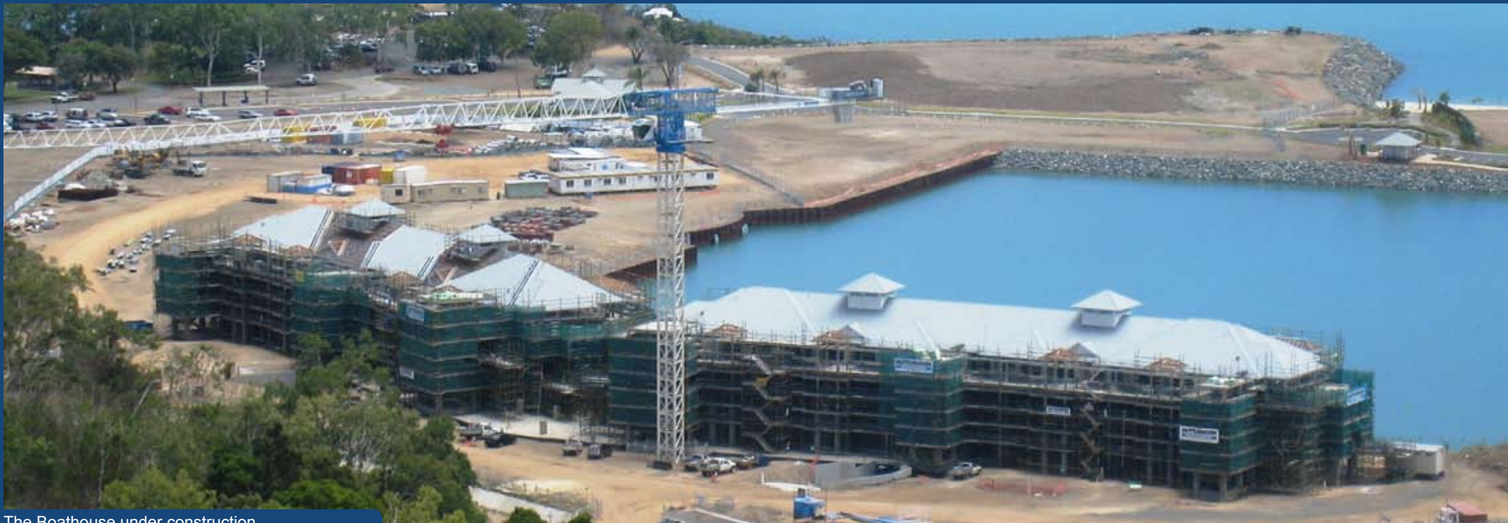
The Boathouse under construction
