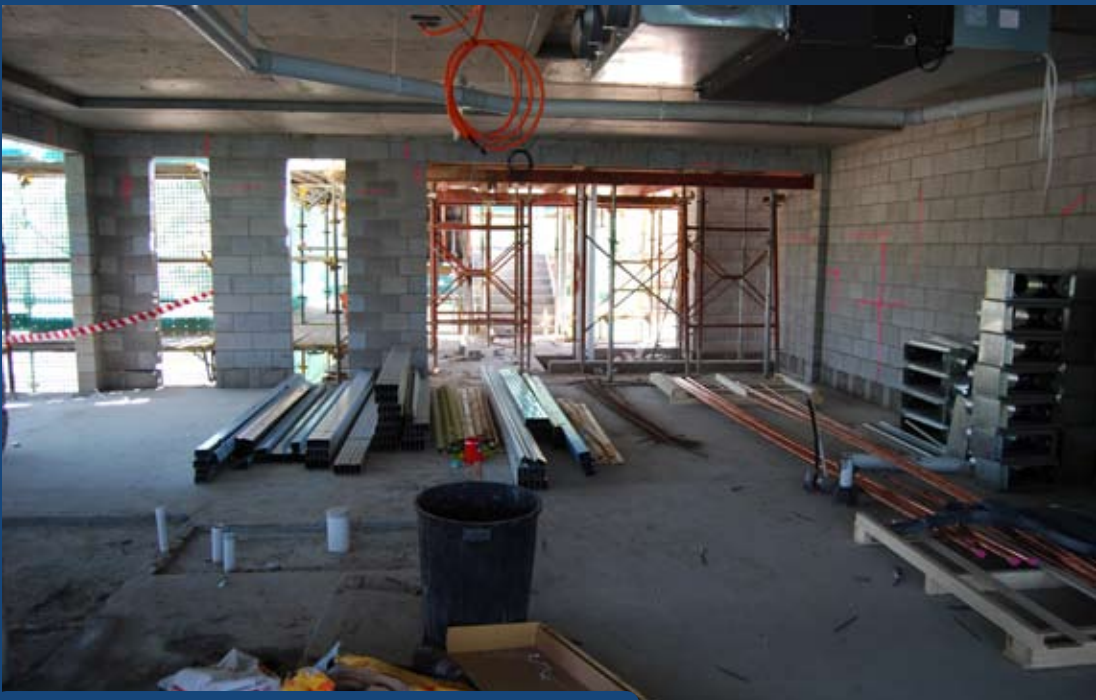
The Boathouse Apartment under construction
