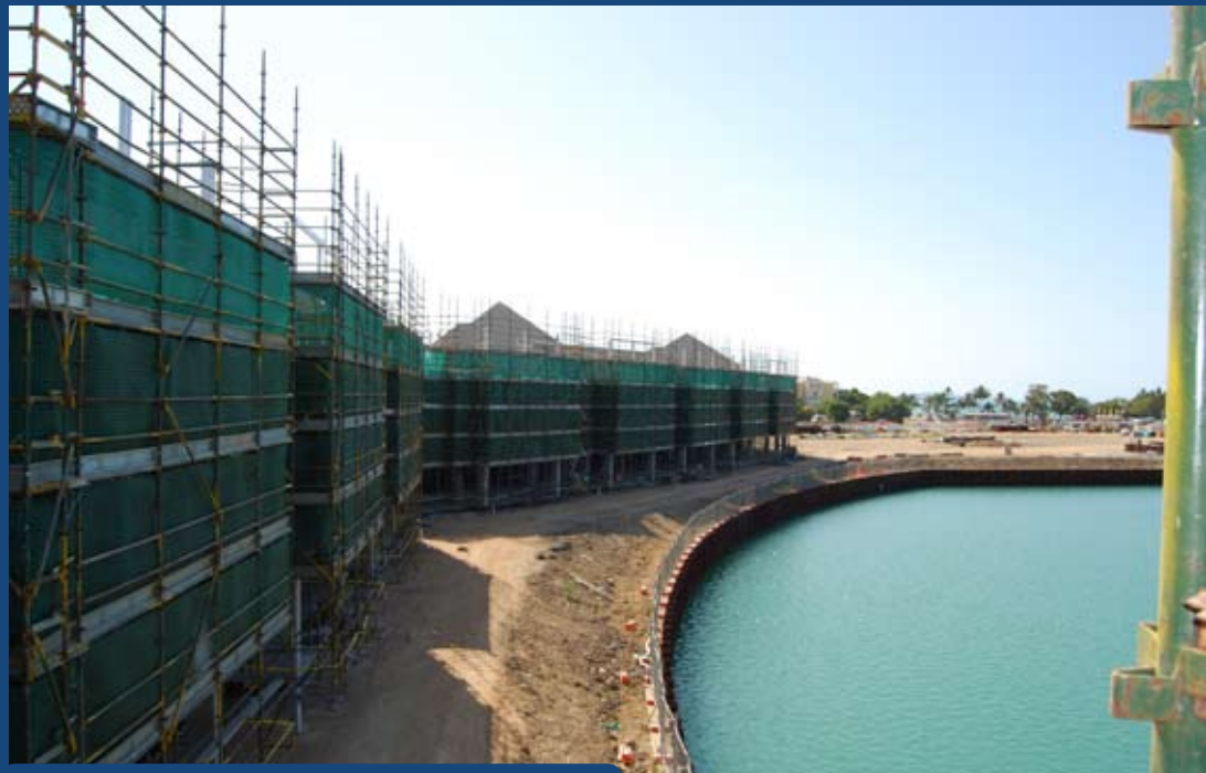
The Boathouse front facade under construction
