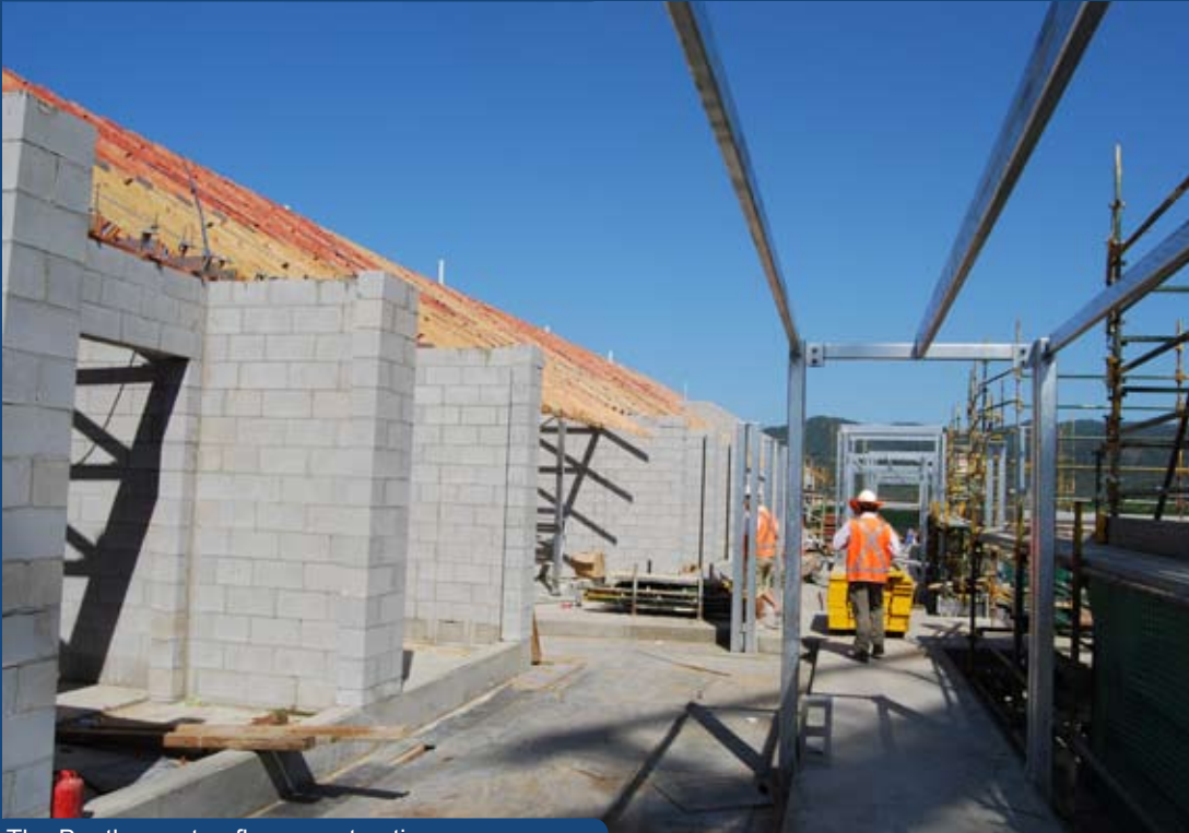
The Boathouse top floor construction
